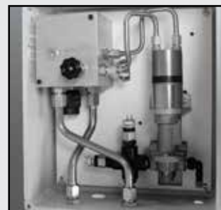
LS102H (Hydraulic Enclosure with Proportioning Valve)
